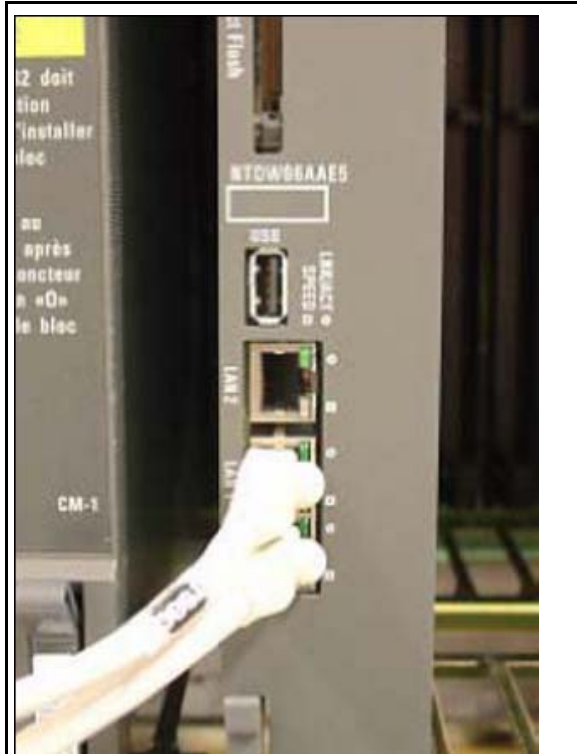
Figure 36 TLAN connection on CP PM faceplate
