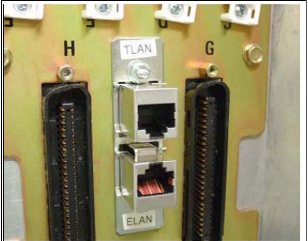
Figure 38 Installed Ethernet port adapter plate
