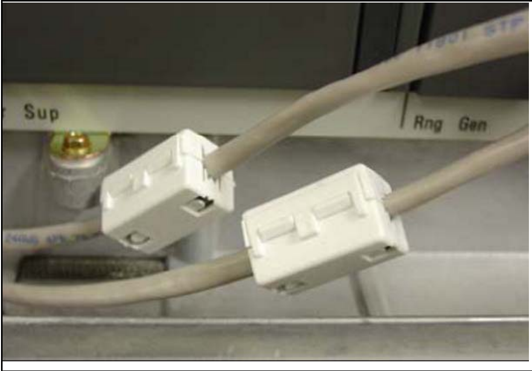
Figure 39 Attached Ethernet patch cable ferrite beads
